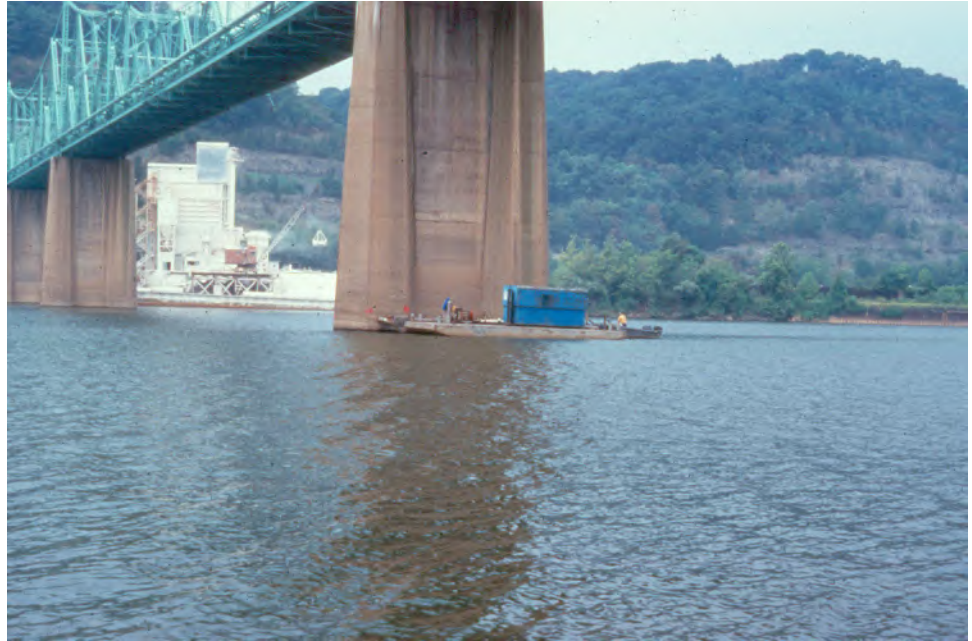
Figure 2.5.6 Inspection Operations from a Barge
