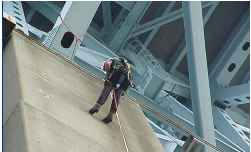
Figure 2.5.9 Inspector Rappelling Substructure Unit
