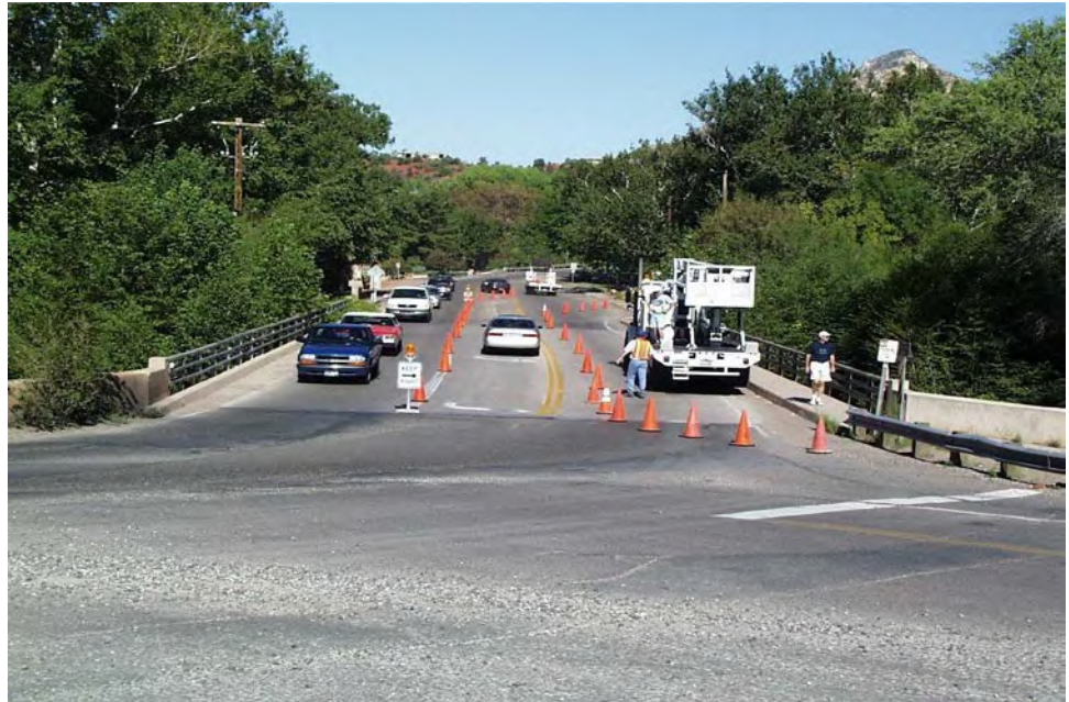
Figure 2.3.1 Temporary Traffic Control Operation
