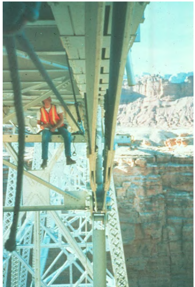
Figure 2.5.4 Rigging for Superstructure Inspection
