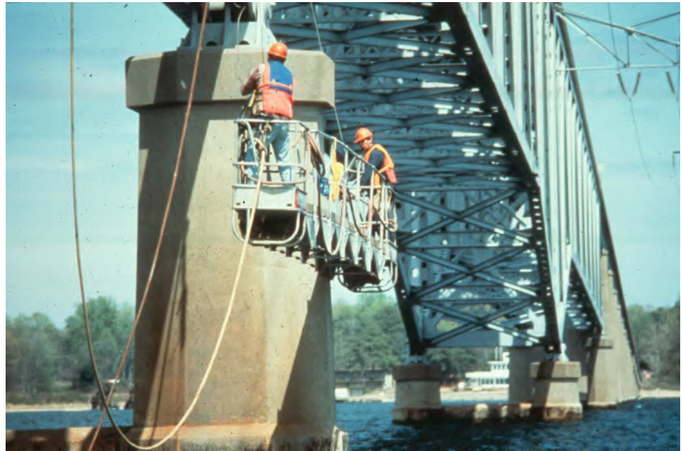
Figure 2.5.3 Rigging for Substructure Inspection
