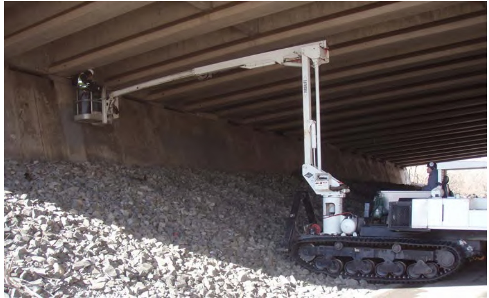
Figure 2.5.19 Track-mounted Man-lift on a Slope
