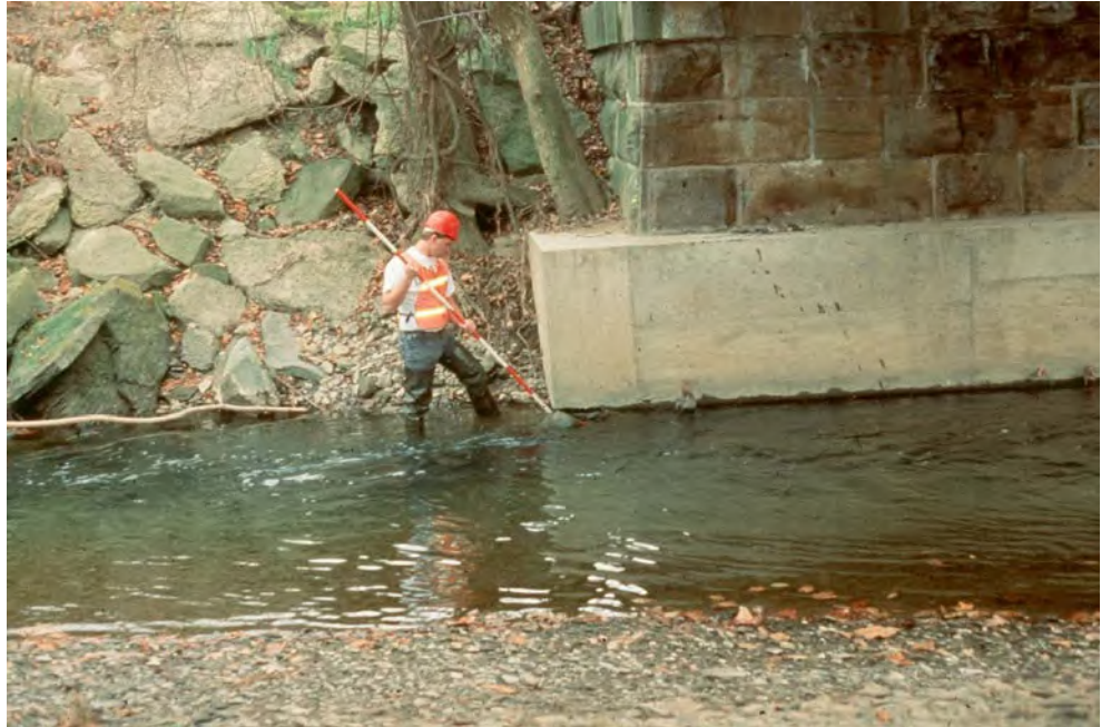
Figure 2.1.5 Inspection for Scour and Undermining
