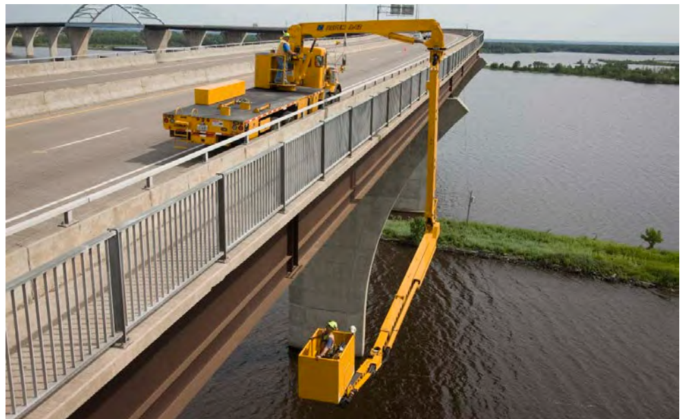
Figure 2.5.20 Under Bridge Inspection Vehicle with Bucket
