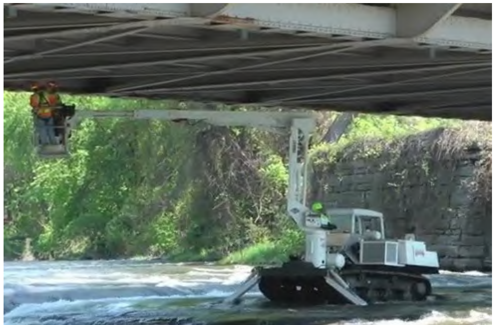
Figure 2.5.18 Track-mounted Man-lift in a Stream
