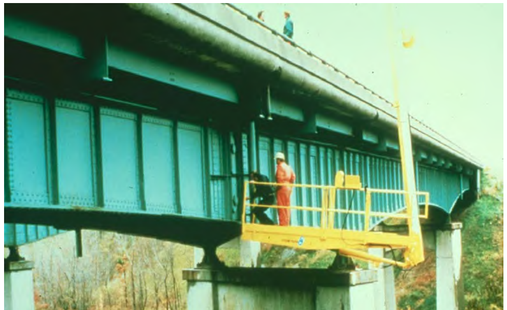
Figure 2.5.21 Under Bridge Inspection Vehicle with Platform
