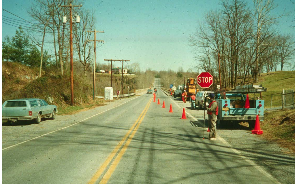
Figure 2.1.4 Temporary Traffic Control Operation
